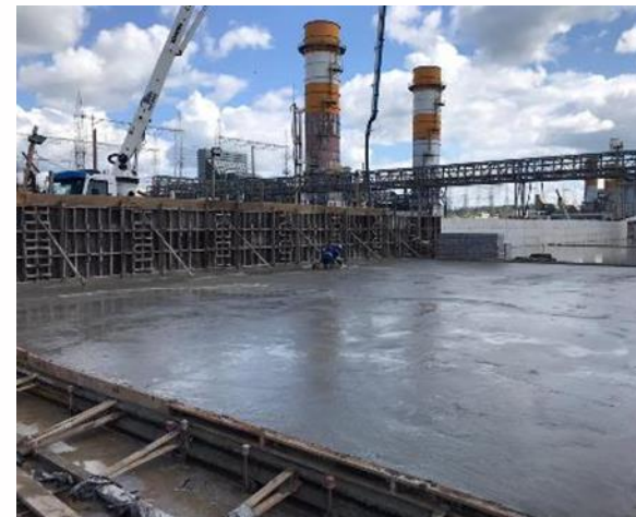
Cooling tower bottom slab
