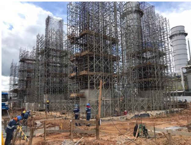
Preparation of the concrete base columns of the steam turbine
