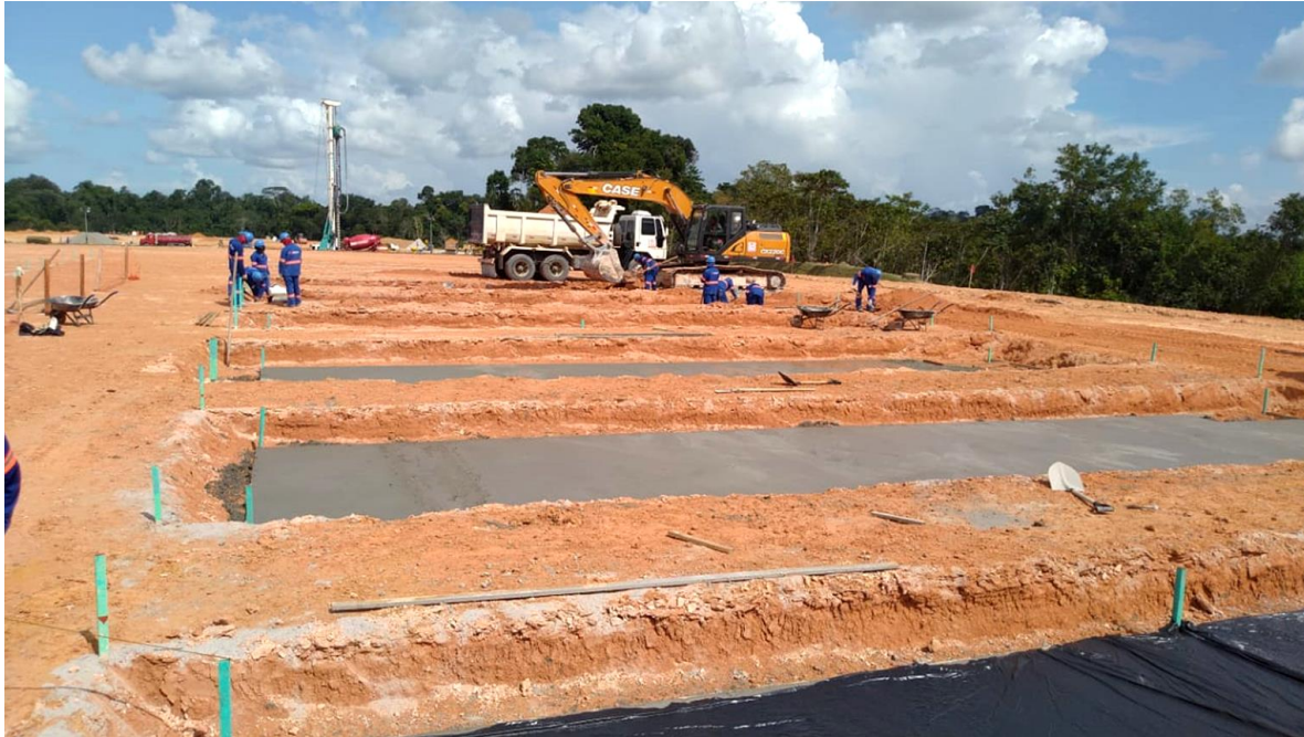
Foundation of cryoboxes
