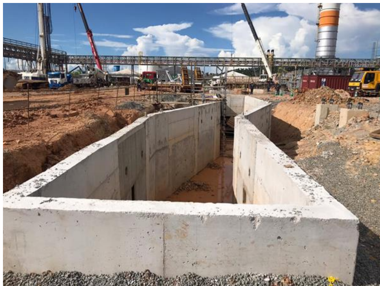
Installation of pre-molded cable galleries
