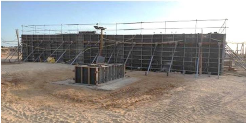
Construction of the steam turbine base
