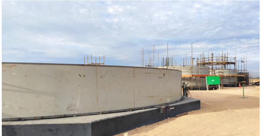
Mounting of water tanks
