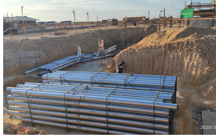
Underground – electrical foundation
