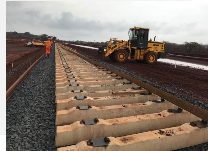
Installation of sleepers – Rio Verde (GO)
