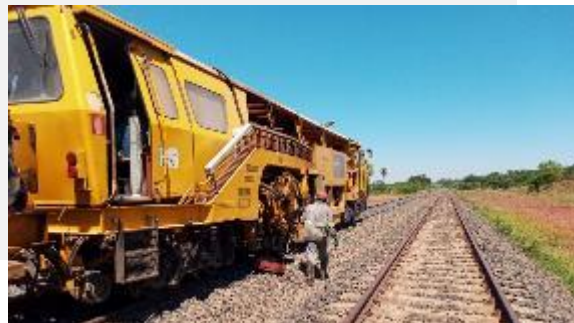
Rail levelling
