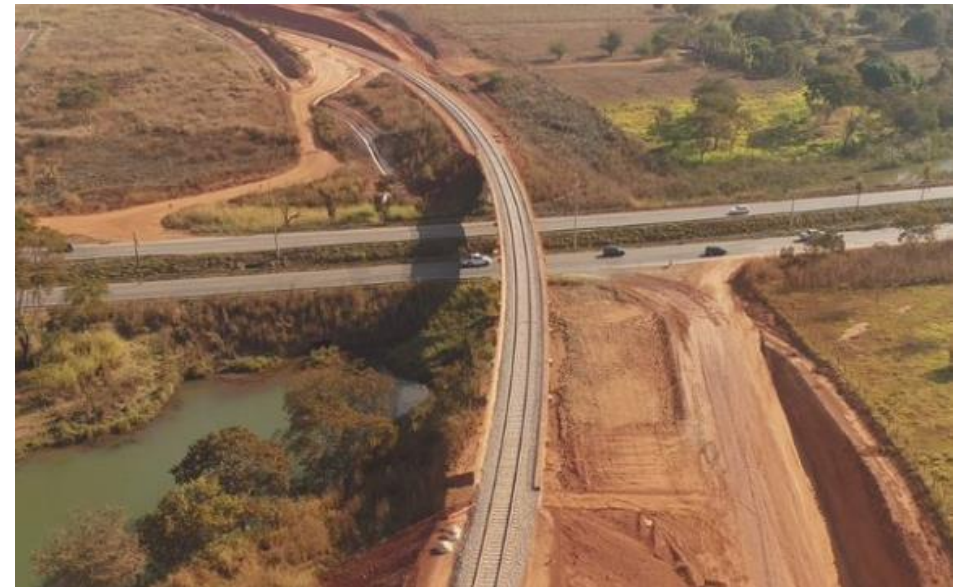
Overpass over GO 070 – km 36 – Goianira/GO
