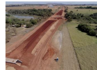
Palmeiras de Goiás/GO Infrastructure services
