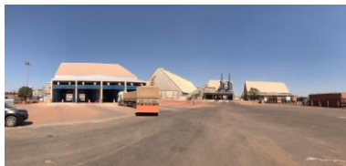
4 new road hoppers More EFFICIENCY for unload Totaling 15 road hoppers
