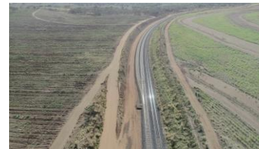
Fernandópolis/SP Connection yard - 5km Central Network and Paulista Network
