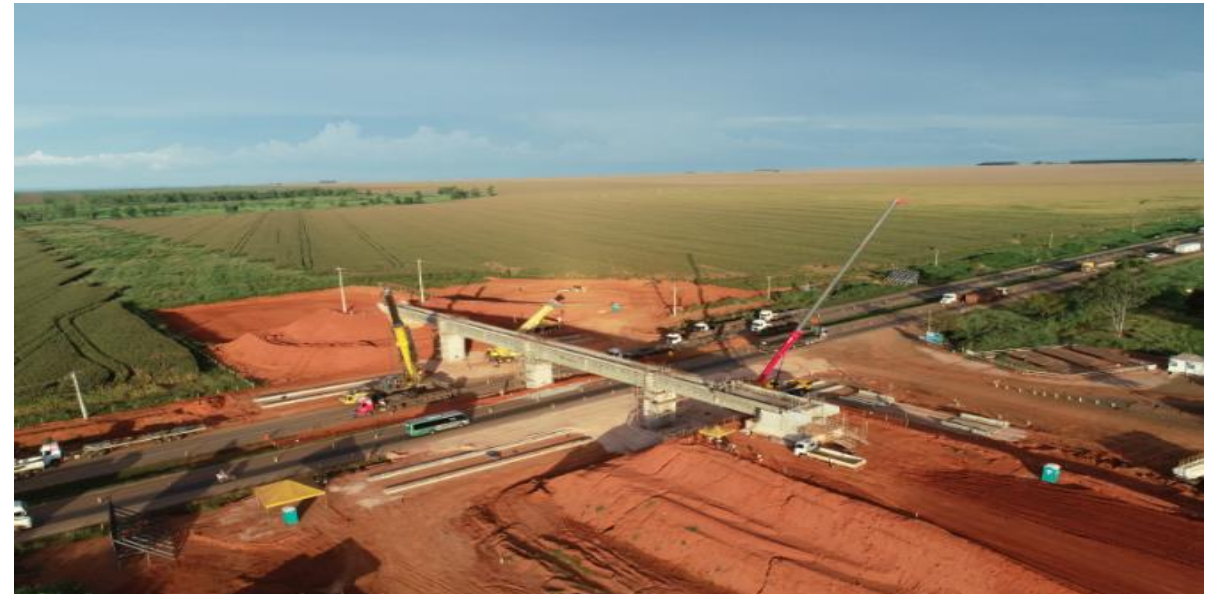
Railroad viaduct crossing BR-163 at the exit of the Rondonópolis
