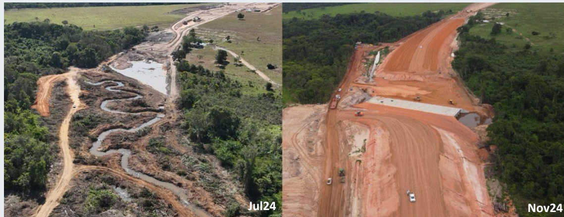
Earthworks in critical sections (km 56)
