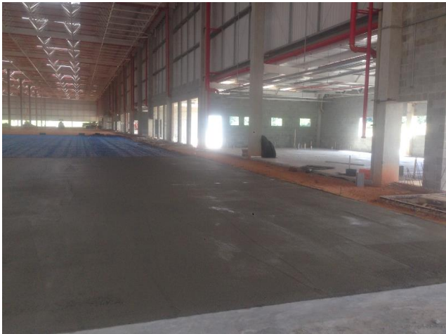
Concretagem de Piso Industrial e Kits.
