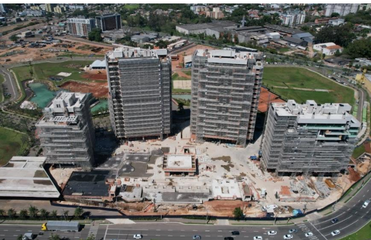
Construction site, Golden Lake phase 1 (Lake Victoria)- Oct-24
