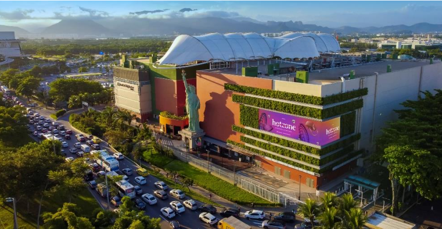
NYCC renovation – Rio de Janeiro, RJ
