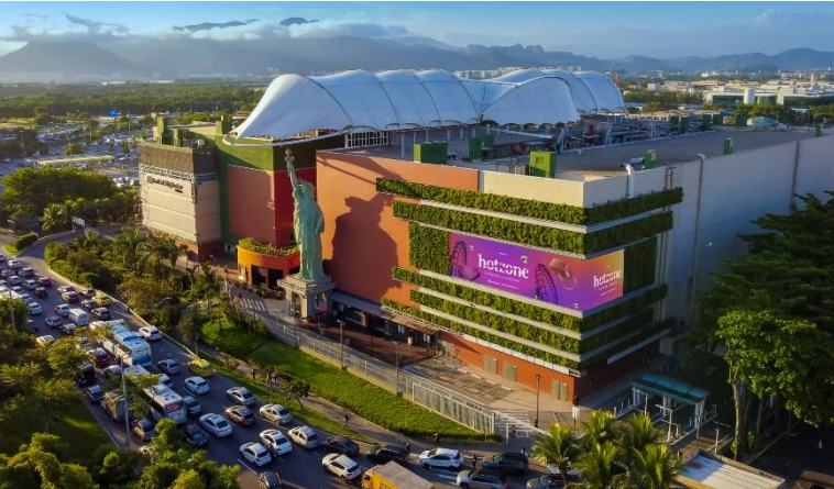
NYCC renovation – Rio de Janeiro, RJ
