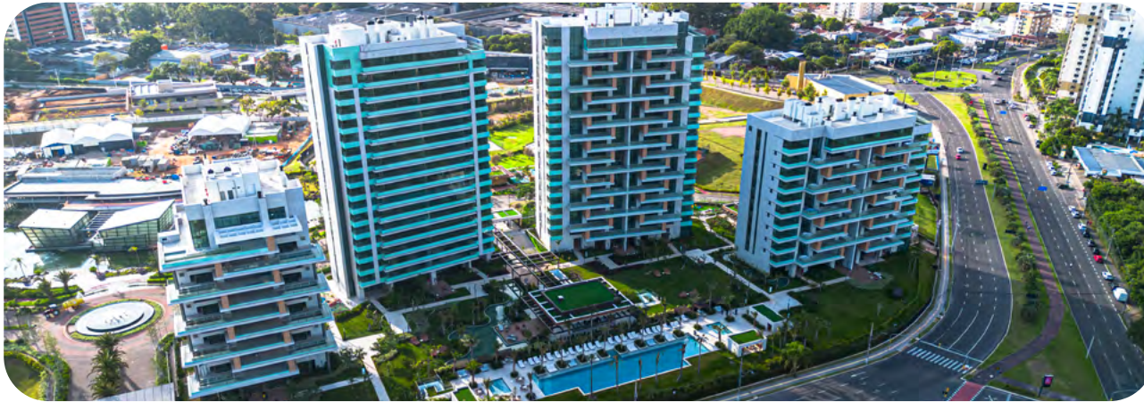
Golden Lake, RS (under construction)
