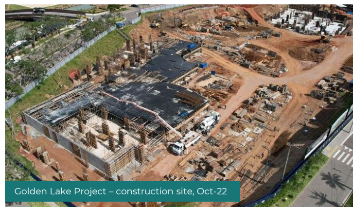
Golden Lake Project – construction site, Oct-22
