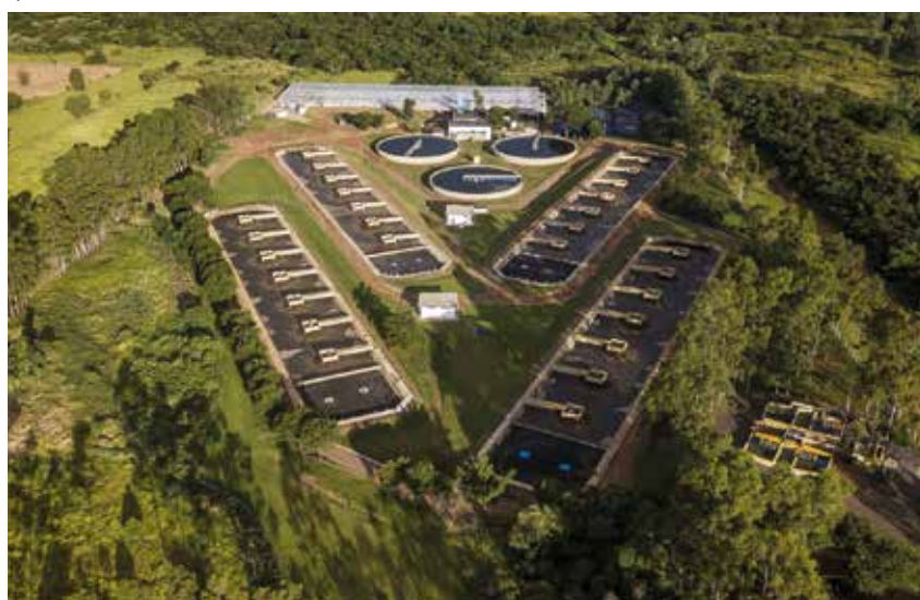
We supported the modernization and expansion of the Baguaçu Sewage Treatment, in Araçatuba (SP) | Photo: Samar Collection
