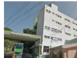
Hospital Unimed ABC
