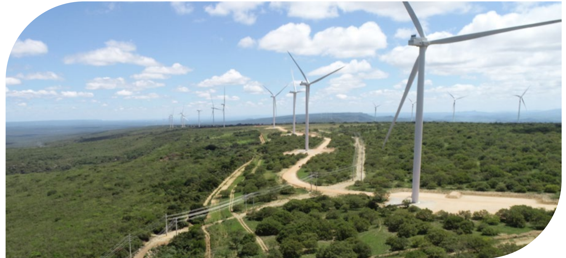
The contract with Enel for wind power supply will serve almost half of the Renner units in the country.
