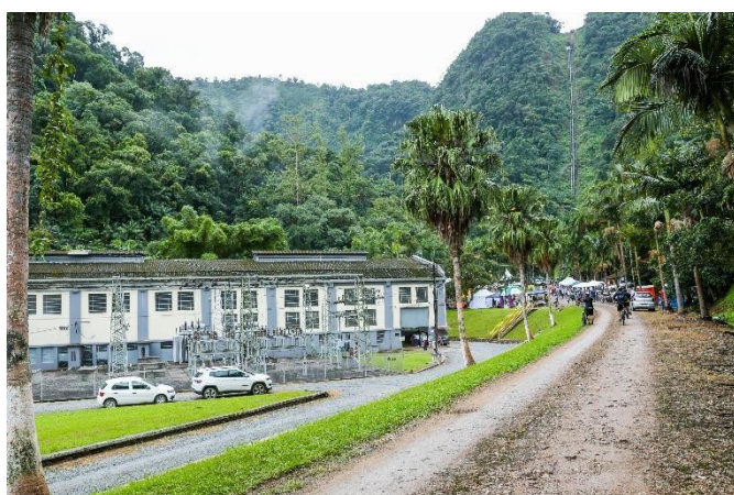
Bracinho Power Plant
