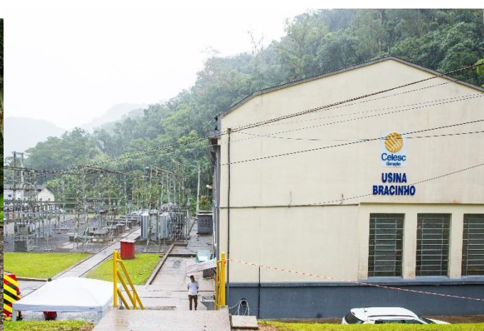
Bracinho Power Plant
