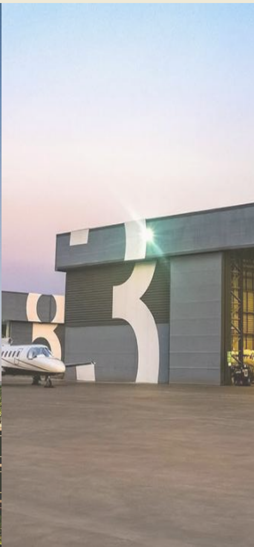
SP Catarina Executive Airport new hangars + apron
