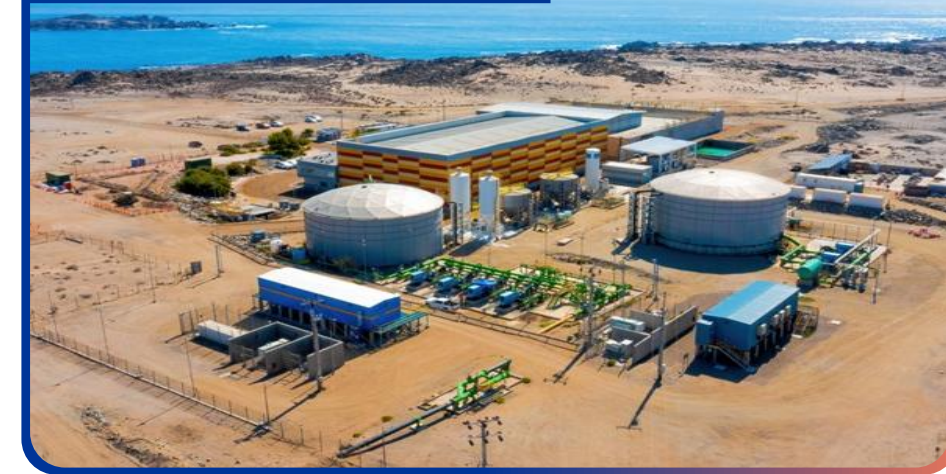
Aguas CAP – Desalination plant
