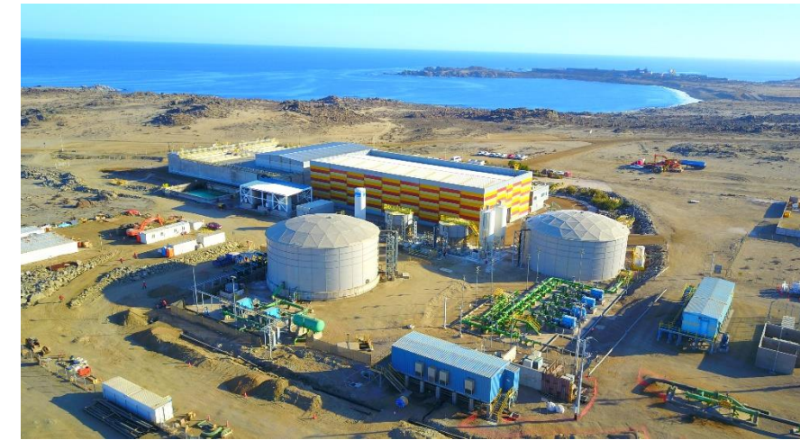
Desalination Plant: Cleanairtech
