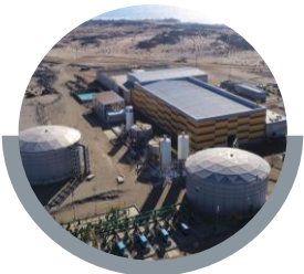
Desalination Plant: Cleanairtech
