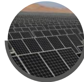
Structures for solar panels
