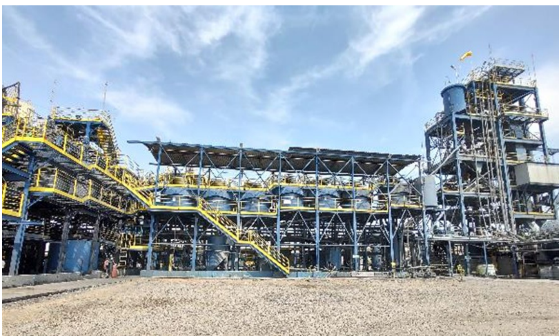
Figure 12-6: Data verification: Processing plant (September 2022)
