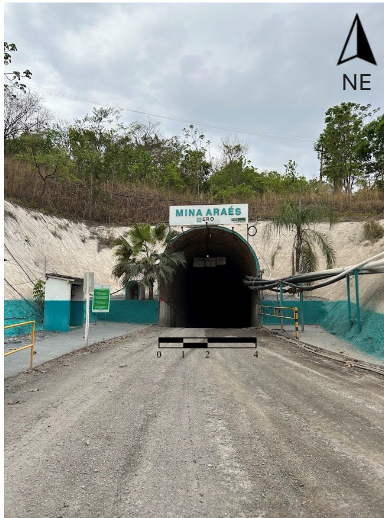
Figure 5-2: Mine Portal (NX Gold, 2024)
