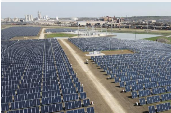
Solar Panels & Midlothian Industrial Unit
