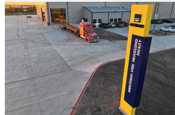
Steel Processing Facility
