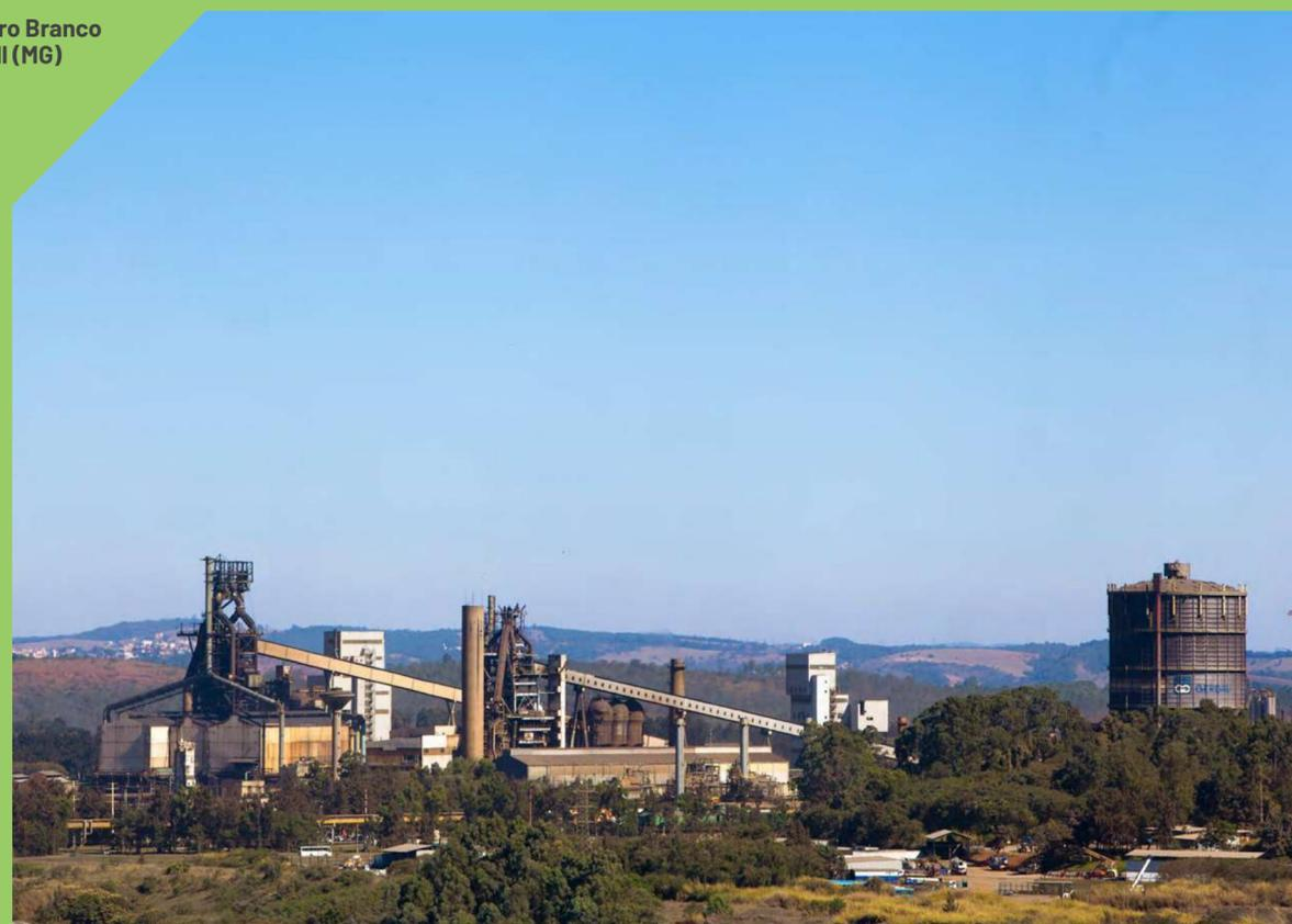
At our Ouro Branco facility we monitor emissions from fixed sources (stacks). Particulate, NOx, SO<sub>2</sub>, and H<sub>2</sub>S are manually monitored depending on the specificities of the process and applicable laws. We continuously monitor the company's main fixed sources of emission. For diffuse or fugitive sources we moisturize, apply polymers, or use mechanized weeping, among others.
