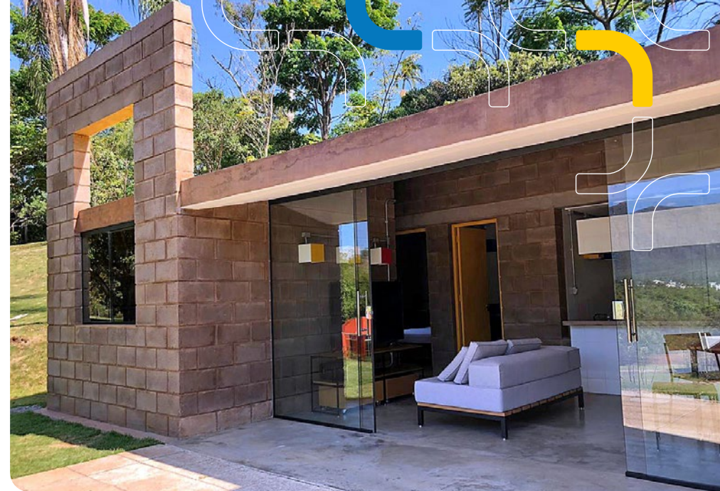
"Sustainable House": house built with Gerdau's dam waste - Gerdau Germinar Biocenter, Ouro Branco (MG)
