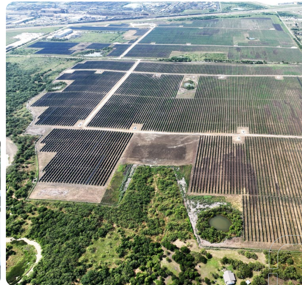
Midlothian solar farm, USA
