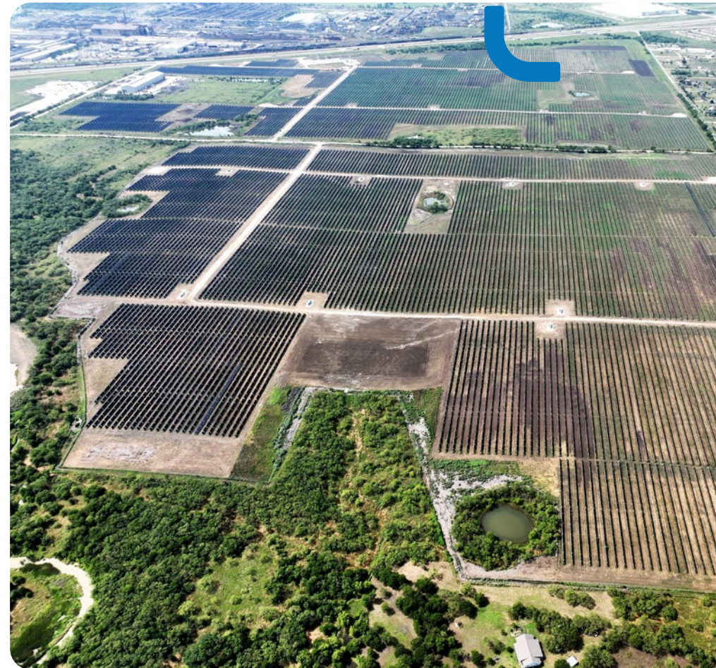
Midlothian solar farm, USA
