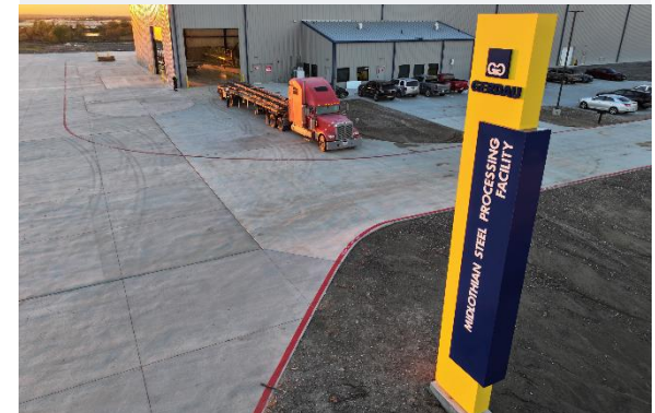
Steel Processing Facility
