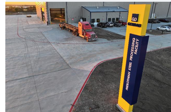
Steel Processing Facility
