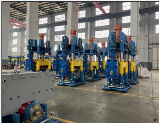
Install of billet handling equipment
