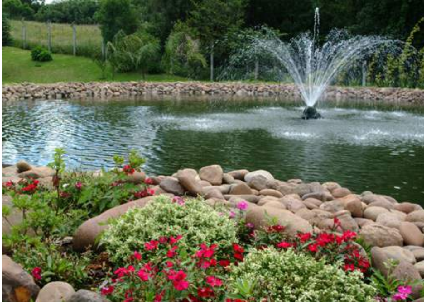
Effluent Treatment Plant – pond treatment step
