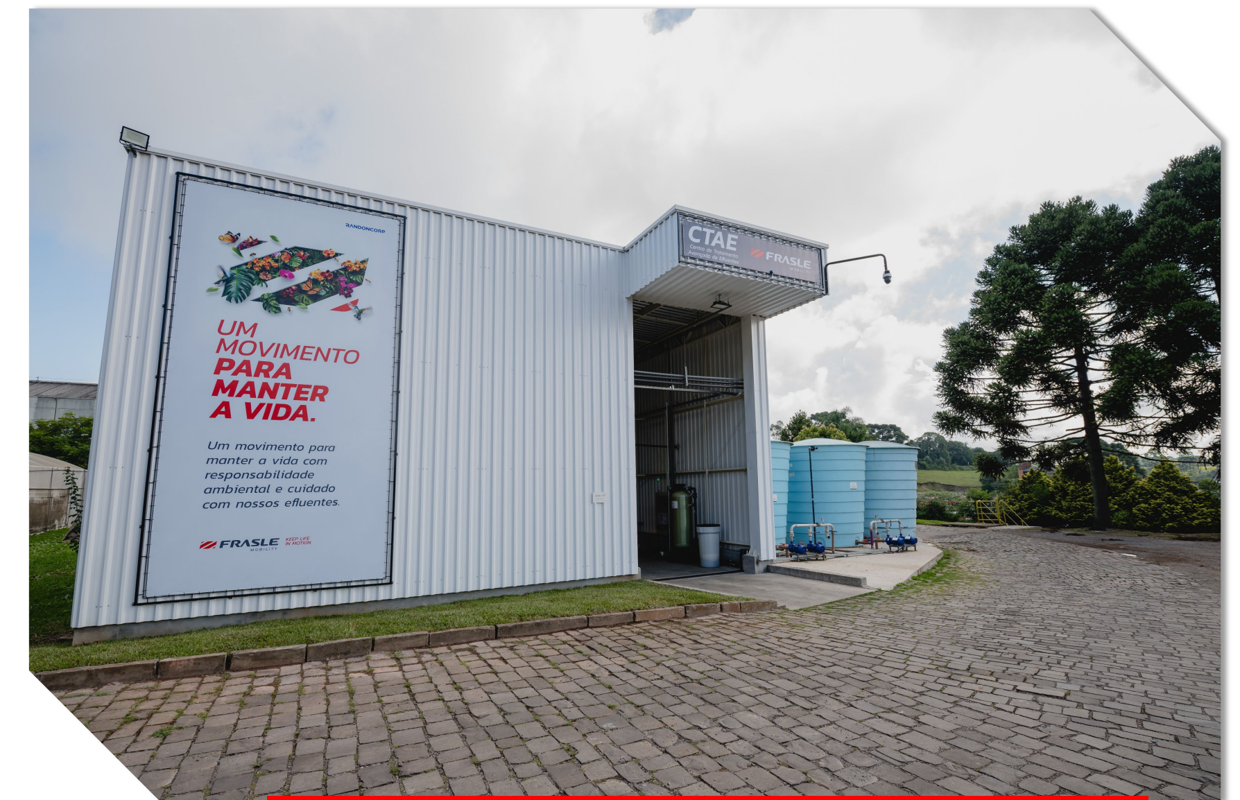
INAUGURATION OF 3 IN-HOUSE SEWAGE TREATMENT PLANTS (STPS)
