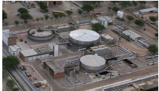
ETE (I, II e III)
