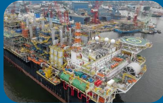
P-78 Module lifting completed
