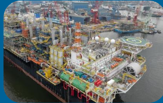
P-78 Module lifting completed
