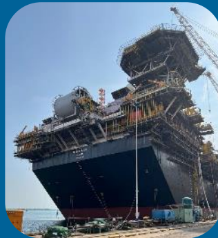
P-80 Start of module lifting Schedule adjustment, changing 1st oil to 2027
