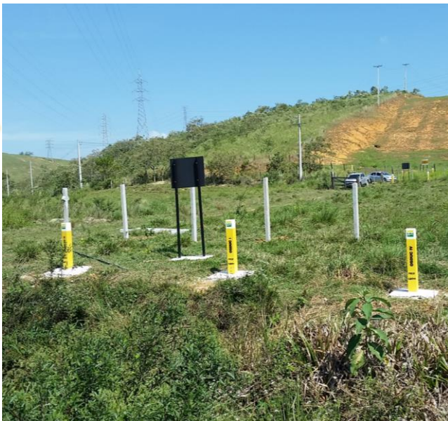
Pipeline land strip located in Rio de Janeiro.
