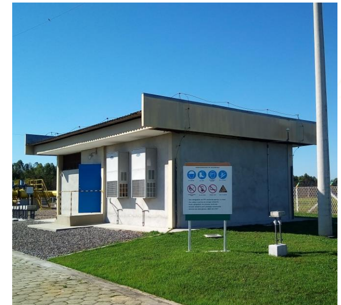
Telecommunication Station located in Espirito Santo.
