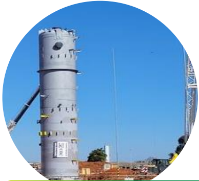
Installation of the vacuum drying tower at REPLAN's new HDT
