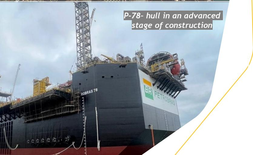
P-78- hull in an advanced stage of construction
