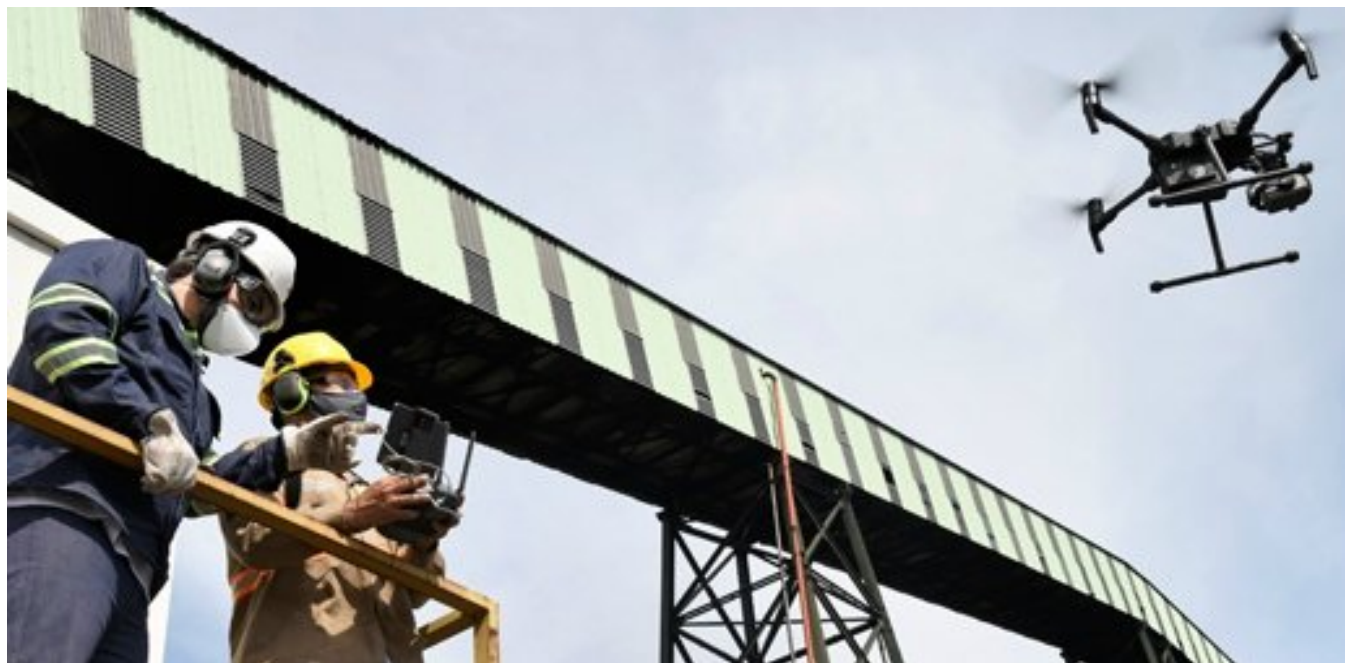
Inspection at height. During 2019, the system autonomously issued 440 maintenance tickets, removing human inspection at 55 roofs.
