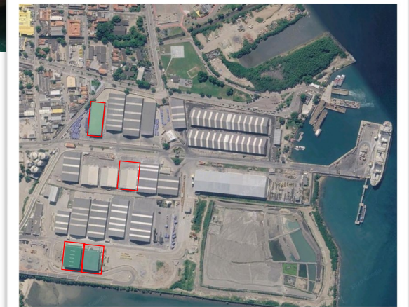
Warehouses operated by Transcopa at the Port of São Sebastião, SP
