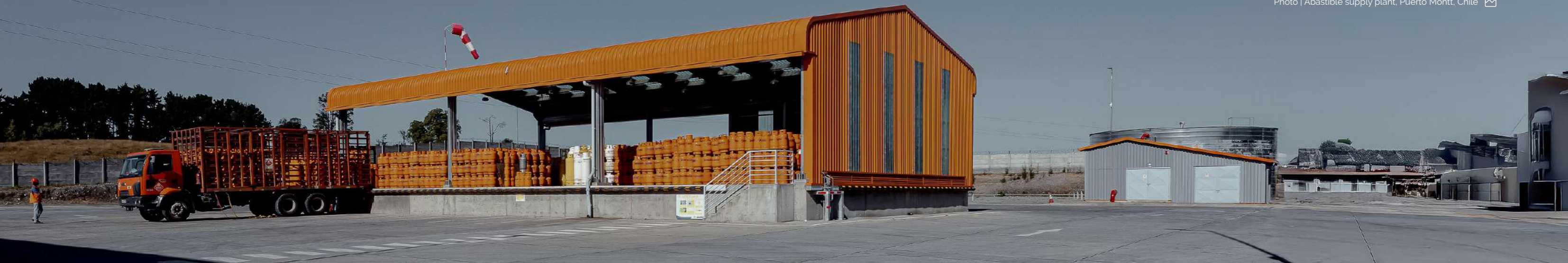
Photo | Abastible supply plant, Puerto Montt, Chile
