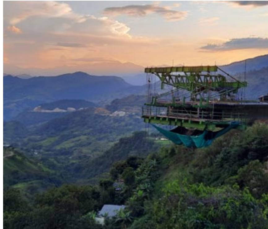
↑ Works of the Guillermo Gaviria Echeverri Tunnel in Antioquia, Colombia
