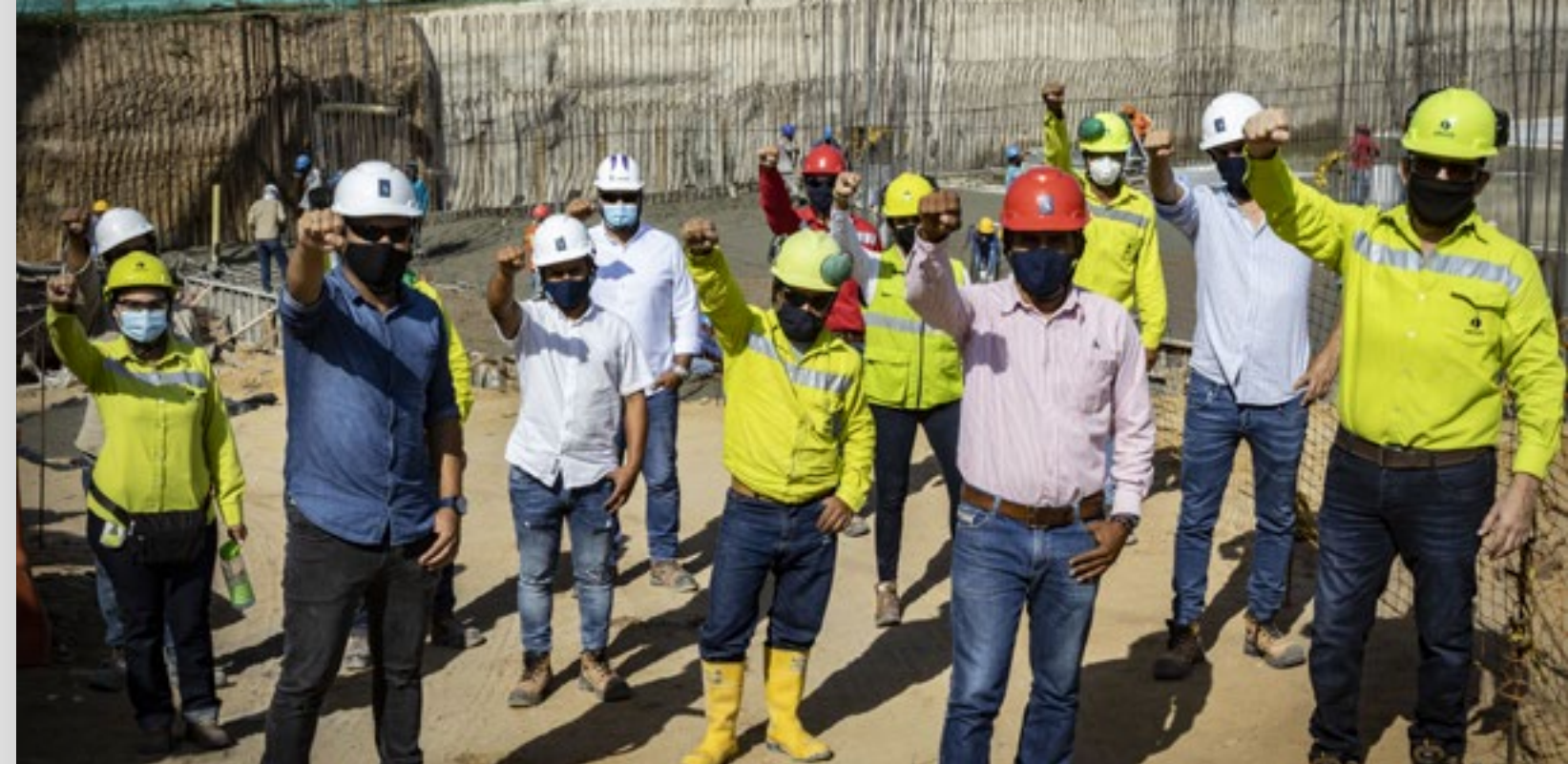
↑ The team in charge of a massive pouring of concrete carried out in Barranquilla, Colombia
