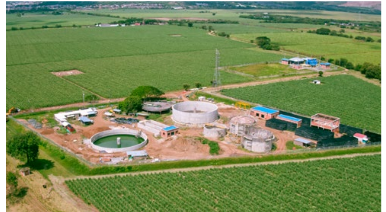
Construction of the wastewater-treatment plant in Valle del Cauca, Colombia
