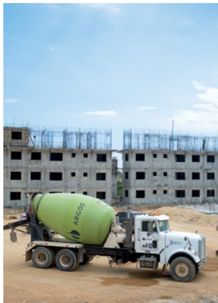
↑ Mixer truck in housing construction project in the Dominican Republic
