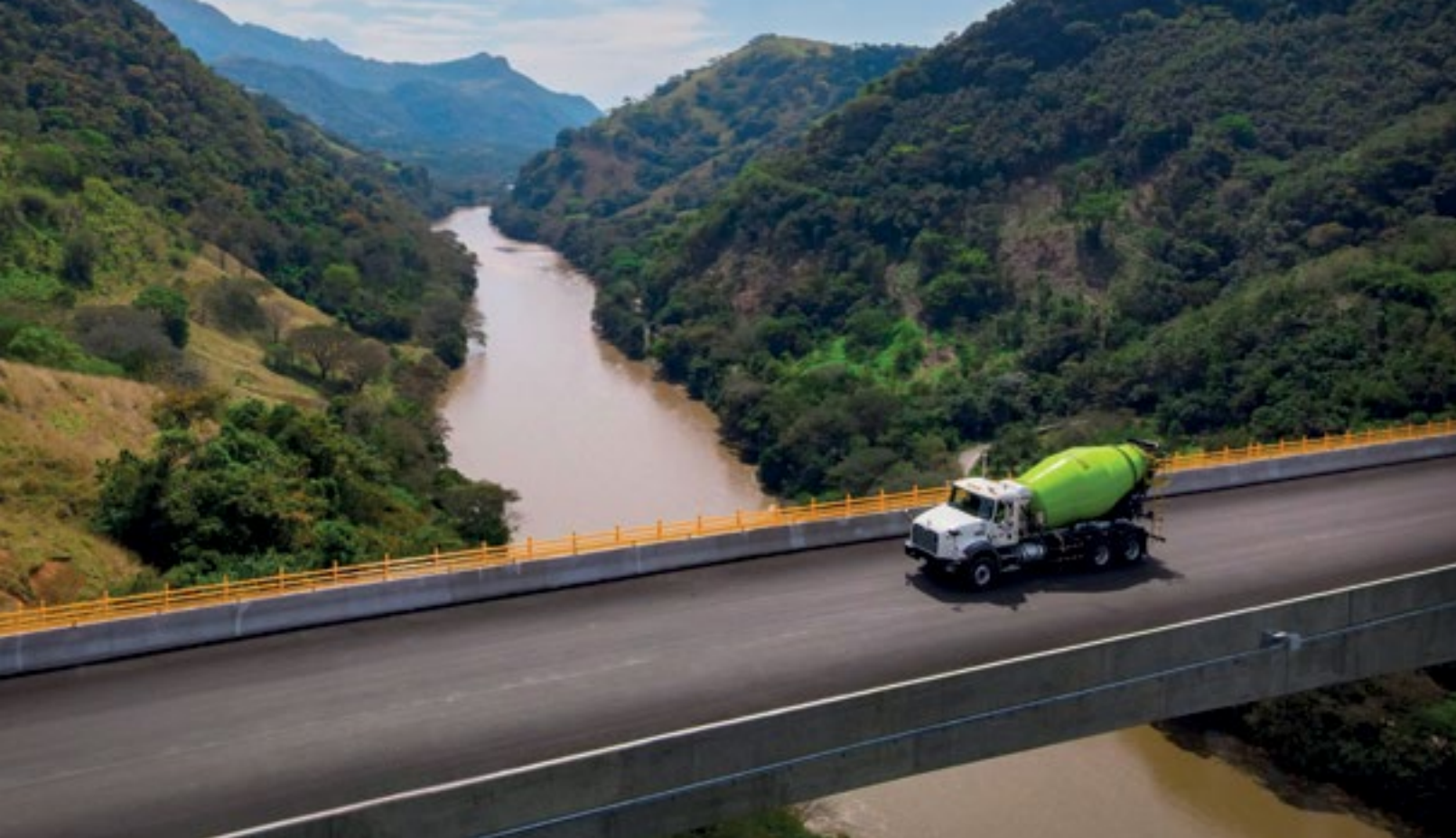
↑ Mixer truck going by the Puente Cauca construction site in Antioquia, Colombia
