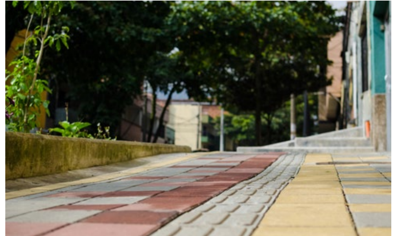
↑ Application of colored concrete on a sidewalk in Medellín, Colombia
