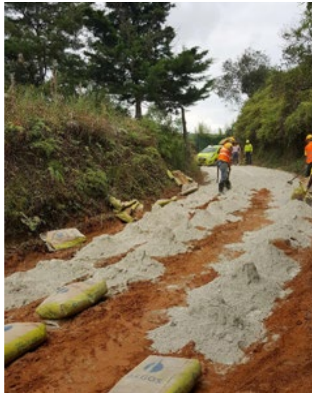
↑ Stabilization of soil through our Vía Forte solution
