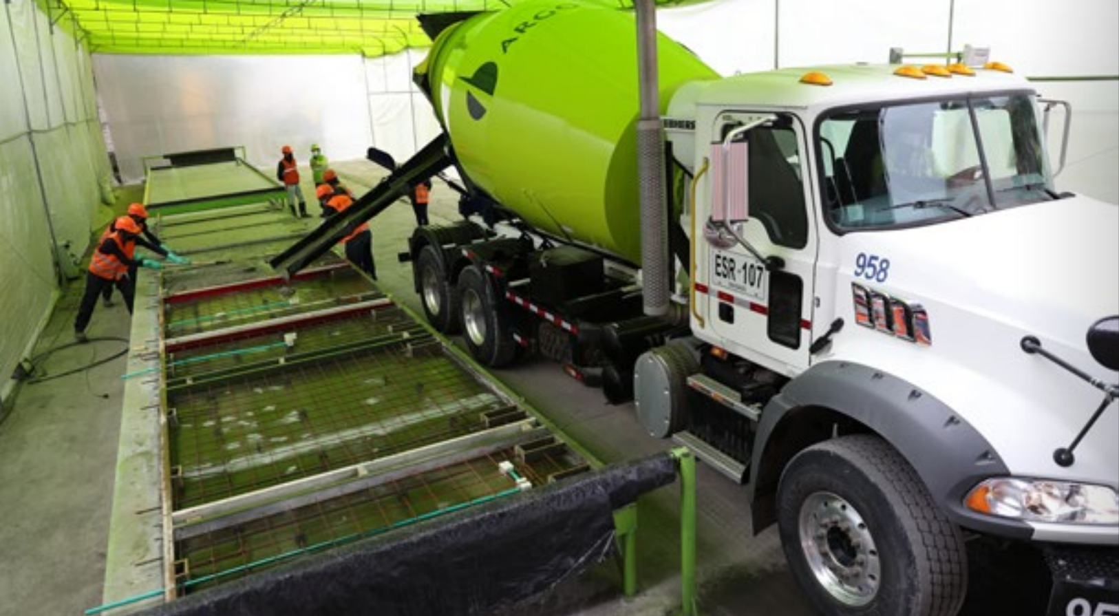
↑ Production of precast concrete modular panels
