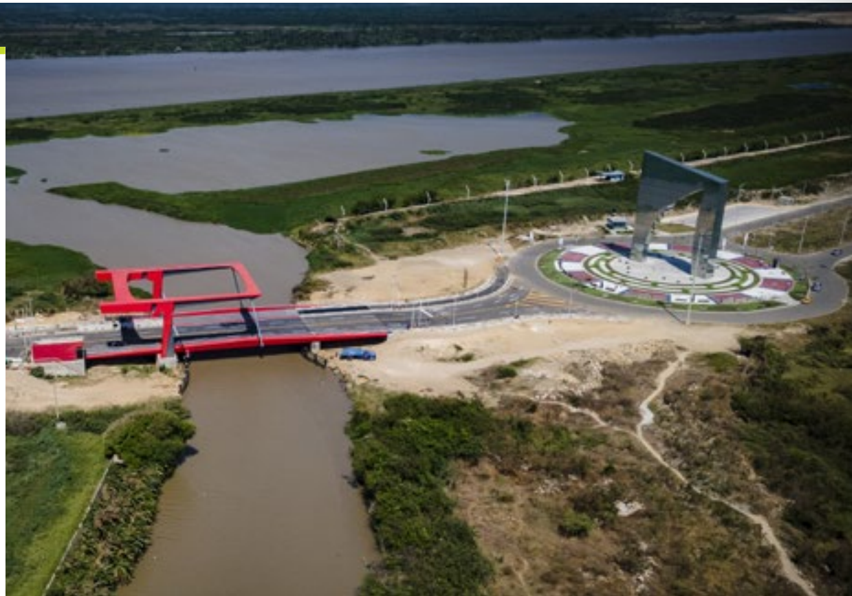
↑ Drawbridge of the Gran Malecón work in Barranquilla, Colombia
