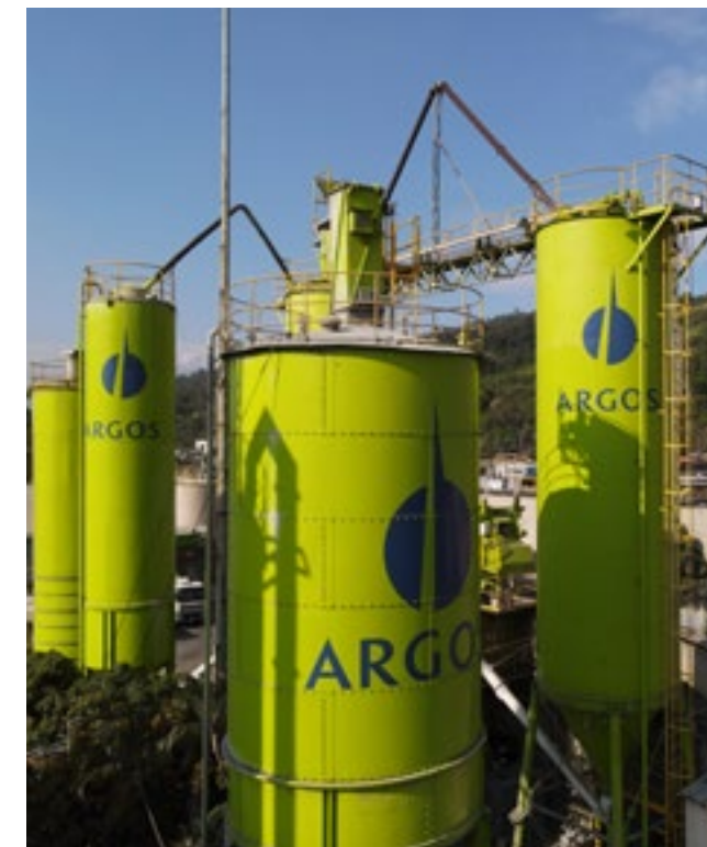
↑ Ready-mix plant in Medellín, Colombia
