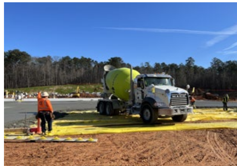
↓ Pouring concrete in Atlanta, the United States
