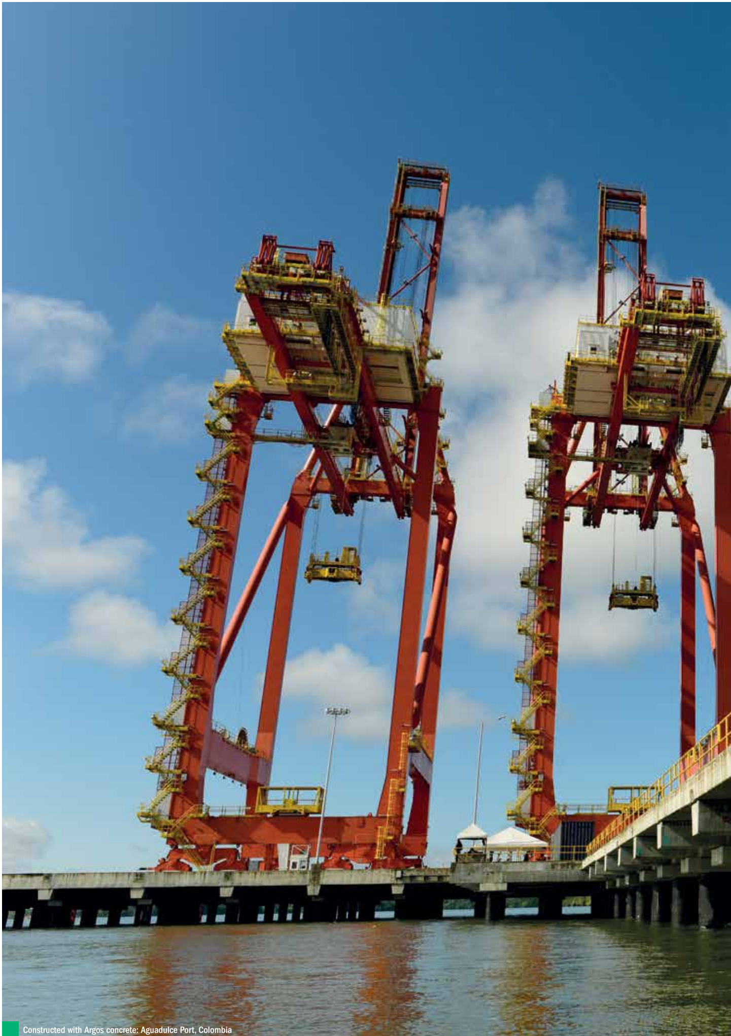
Constructed with Argos concrete: Aguadulce Port, Colombia
