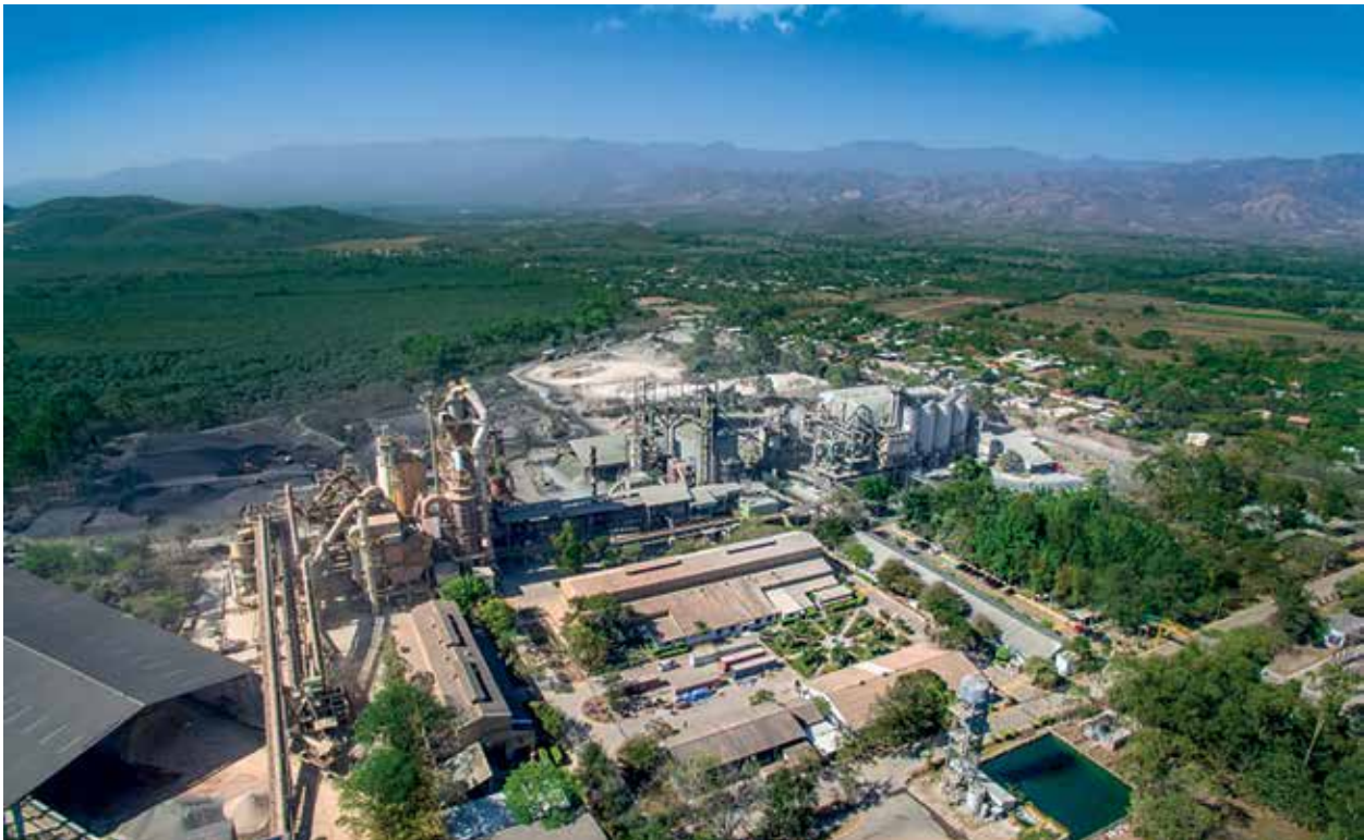
Comayagua Plant, Honduras, Caribbean and Central America
