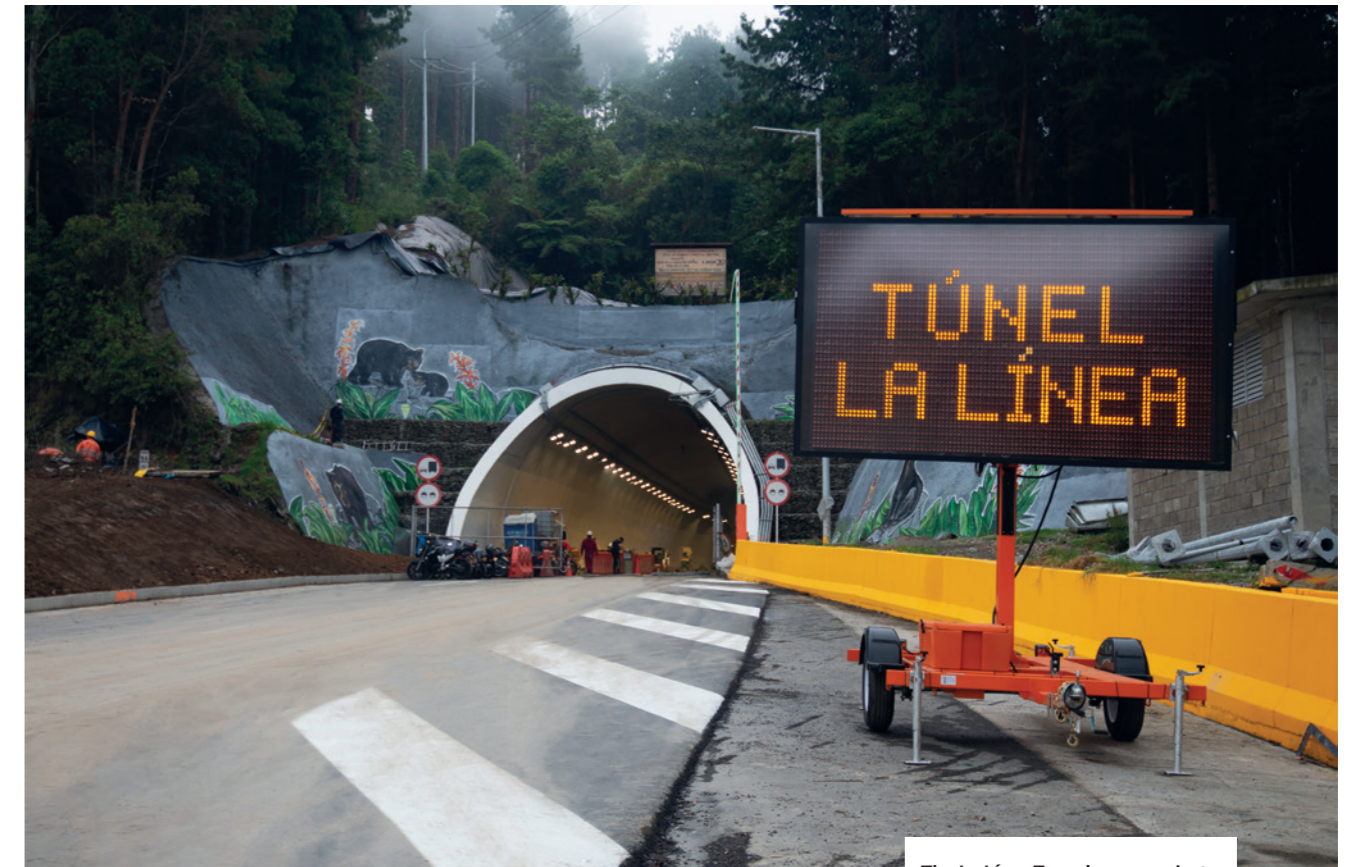
The La Línea Tunnel was a project with great logistic and technical challenges that were met by Argos.
