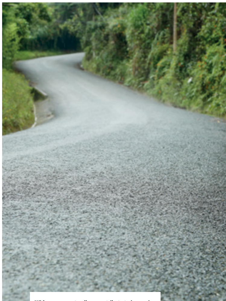
With our cement soil we contribute to improving and building tertiary roads to bring agricultural production centers closer to those of consumption.
