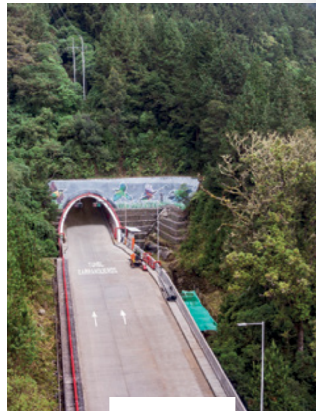
La Linea Tunnel, Colombia, a project with the #ArgosSeal
