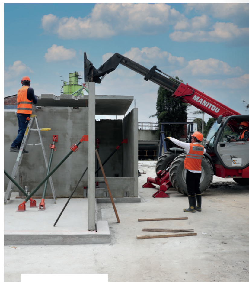
New concrete modular system, Colombia
