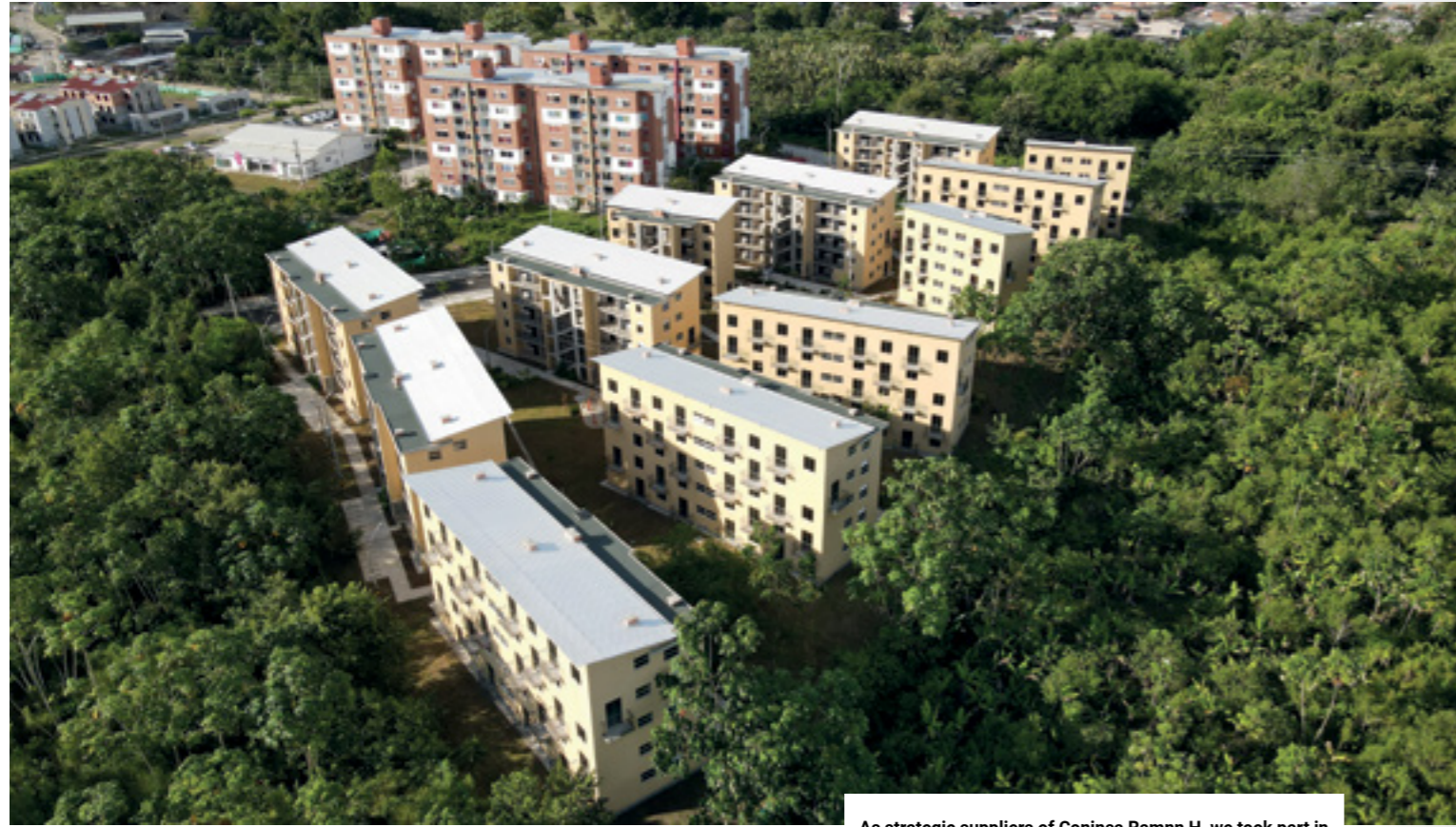
As strategic suppliers of Coninsa Ramn H, we took part in the construction of Curazaos, a social housing project from Comfama that was developed in Apartado (Uraba), Colombia, and which was granted the Habitat Quality award by Minurvi.
