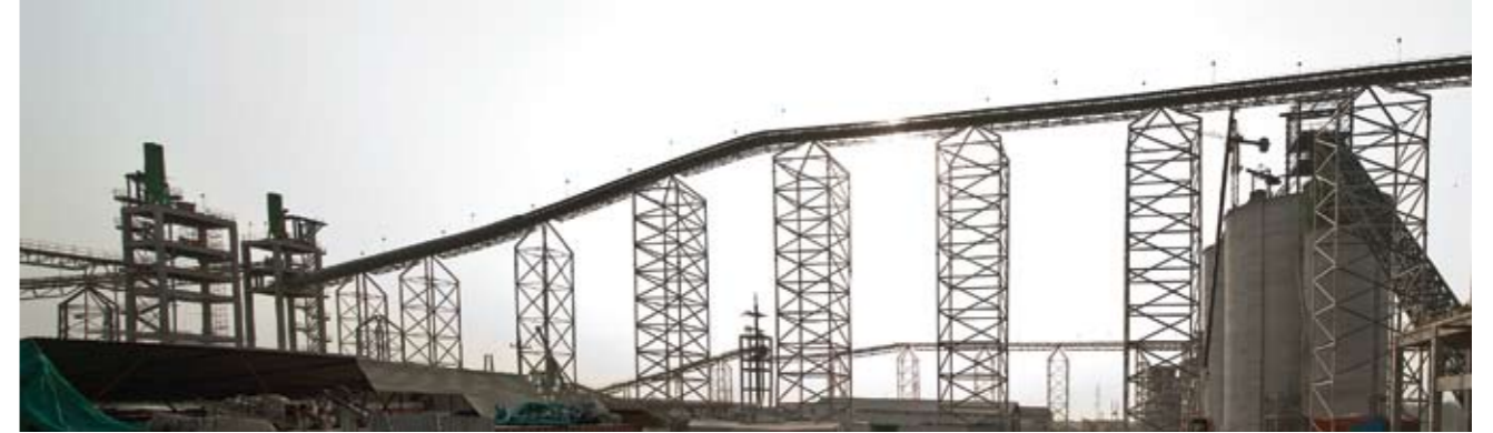
Coal transport Line 4 Cartagena Plant
