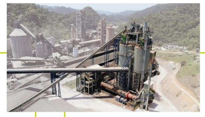
In this process, Clinker use is reduced thanks to the incorporation of calcined clays (artificial pozzolans)
