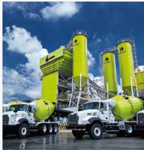
Concrete plant in Panama, Caribbean and Central American Regional Division
