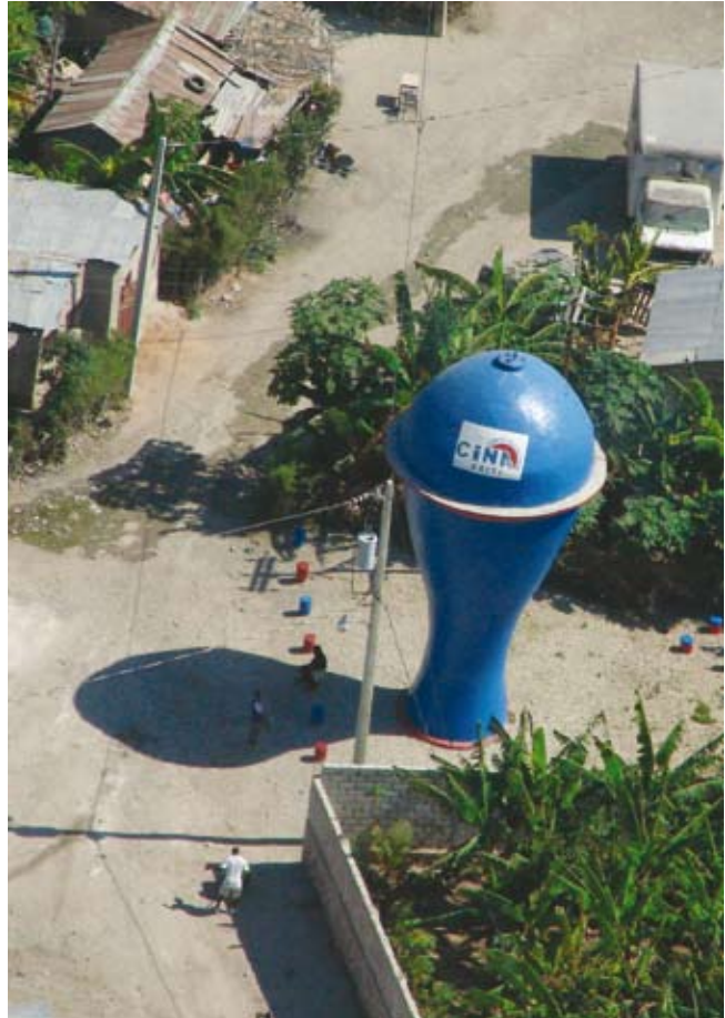
Tanque en Source Metals, Haiti
