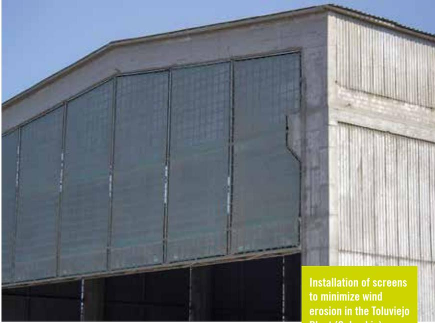
Installation of screens to minimize wind erosion in the Toluvejo Plant (Colombia)
