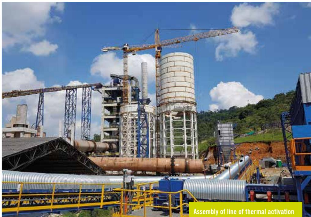
Assembly of line of thermal activation of clays, Rioclaro Plant (Colombia)
