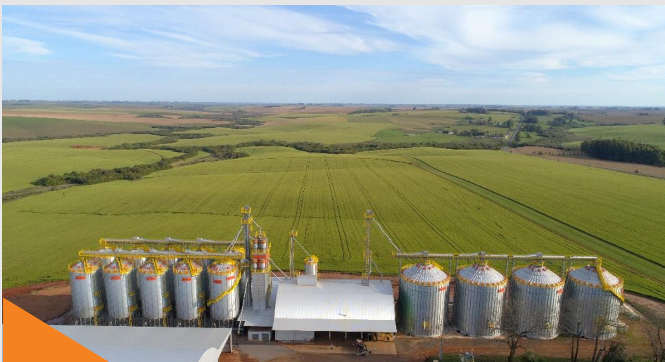
Cruz Alta, in Rio Grande do Sul | Delivered in September 2018 Stored : Soy, Corn and Wheat
