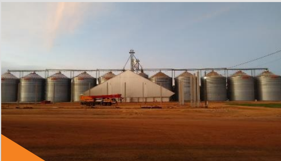
Uruçuí, in Piauí | Delivered in February 2022 Stored: Soy and Corn
