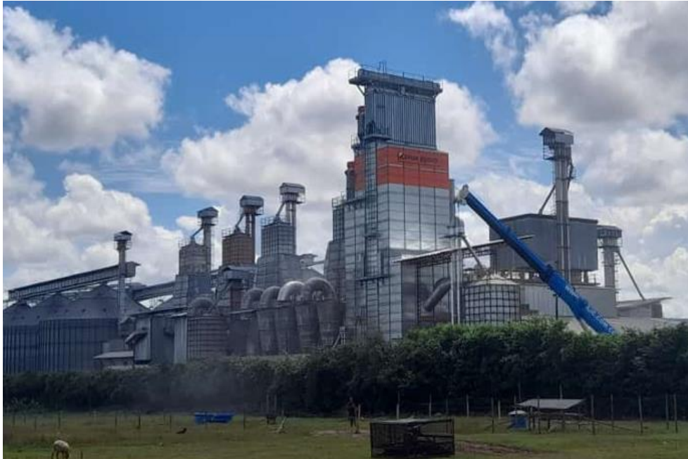
Dryer | Capacity for 3.8 thousand rice bags
