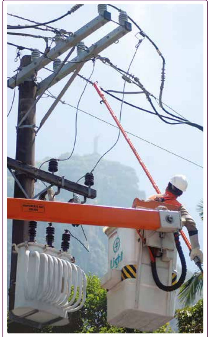
Electrician at overhead network
