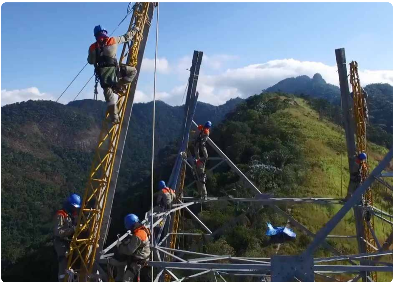
Construction of the Jacarepaguá / Curicica transmission line
