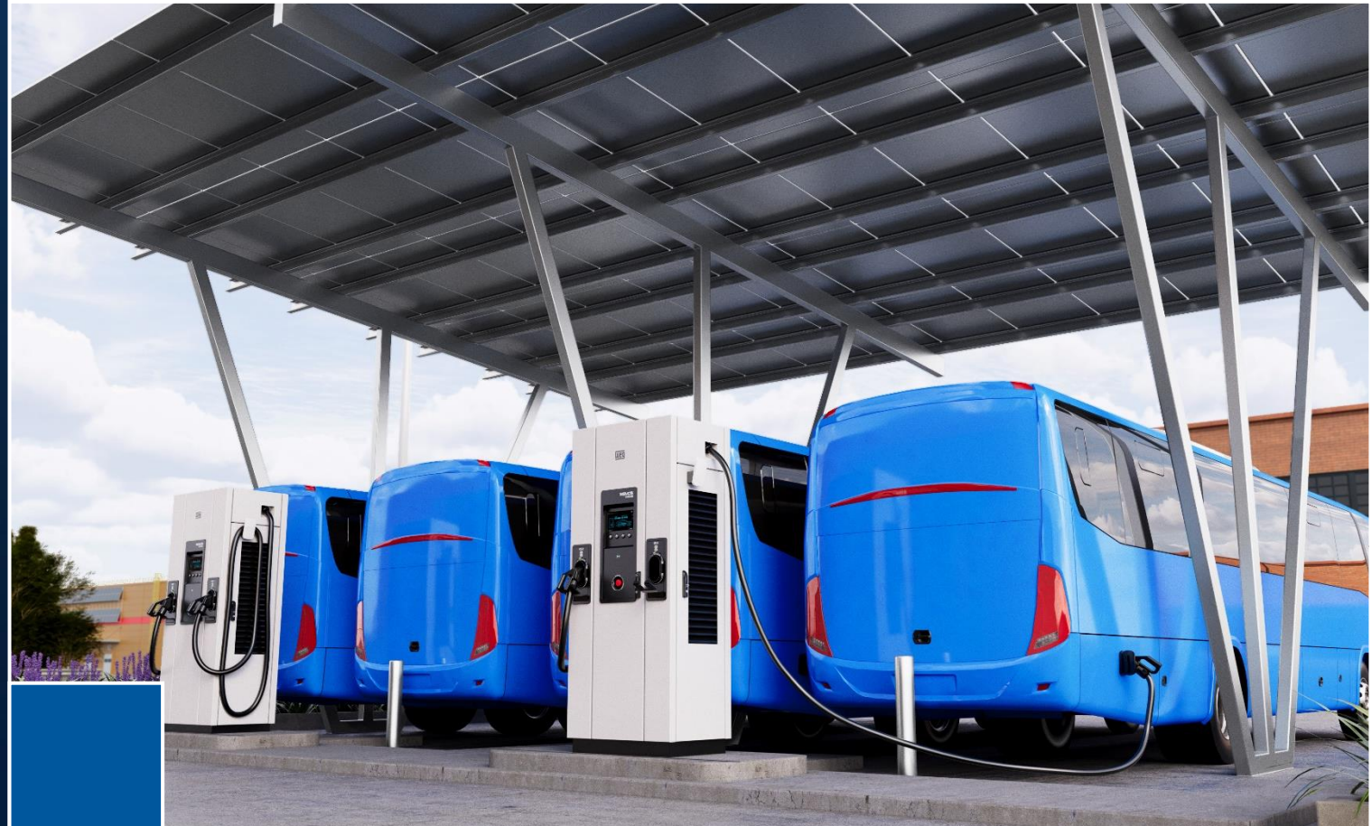
Garages and distribution center
